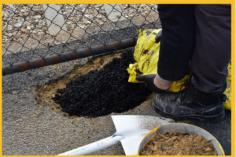
Place PAR in hole in layers of 3 inches at a time and 2. tamp the area until firm. The last layer of PAR is to be 25% higher than the finished level.
